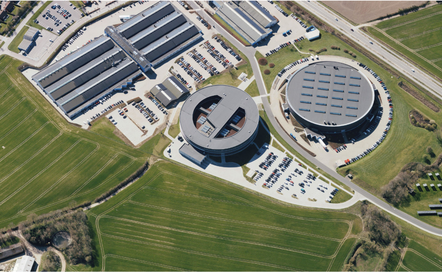
LINAK Headquarters in Guderup, Denmark
